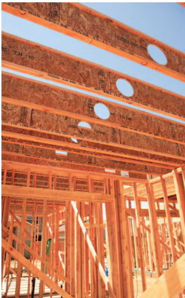
SOFTWARE for design and fabrication enables dealers to pre-cut holes in joists, saving builders' time on the jobsite.
